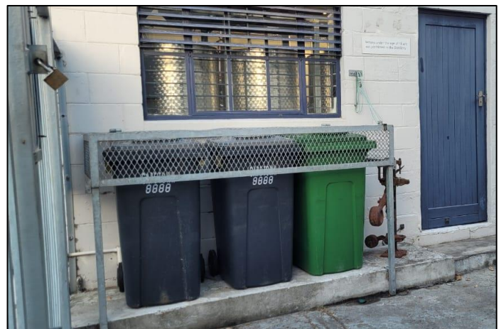
Figure 9. Baboon-proof bin housing at Deep South Distillery.
