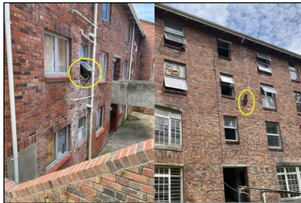
Figure 12. Baboons accessing rooms at Waterfall Barracks.
