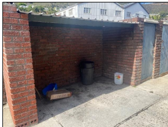
Figure 13. One of the areas identified at West Yard that can be modified to serve as a bin enclosure.
